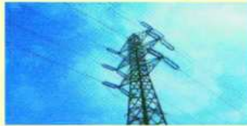
Electricity and Water Connection are Provided
